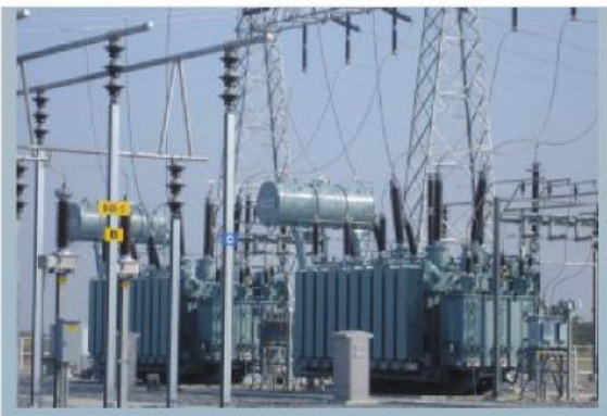
■ 120/160/200 MVA 230 - 121-22 kV Electricity Generating Authority of Thailand
